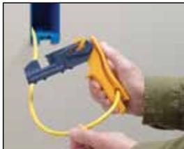
1. Strip cable jacket with a standard cable stripper or the built-in cable stripper.
